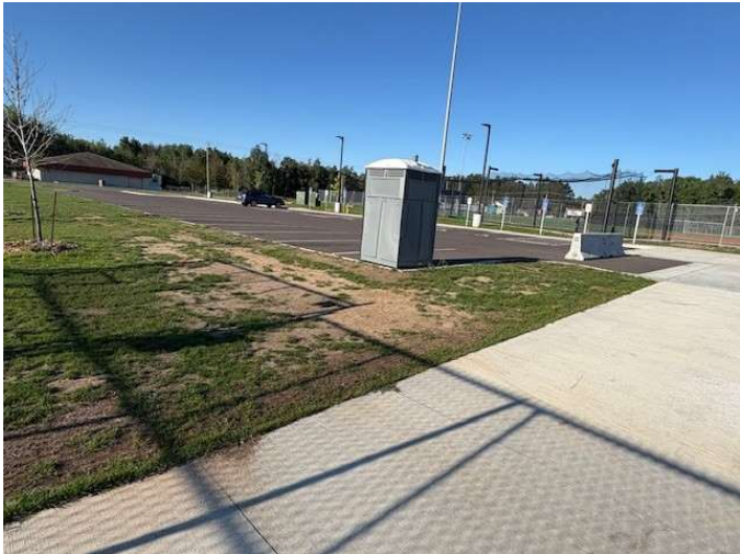
AREA 23 – REPLACE WITH SOD
