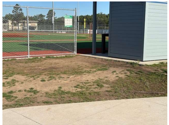
AREA 2 – REPLACE WITH CONCRETE
