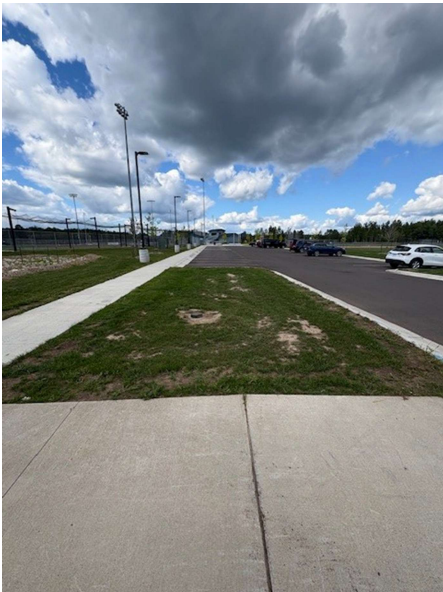
AREA 24 – REPLACE WITH SOD
