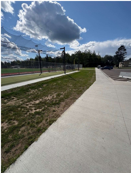
AREA 9 – REPLACE WITH SOD
