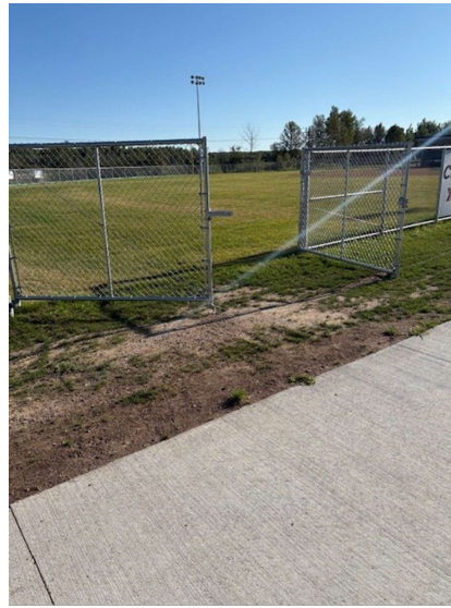
AREA 13 –CONCRETEAT GATE
