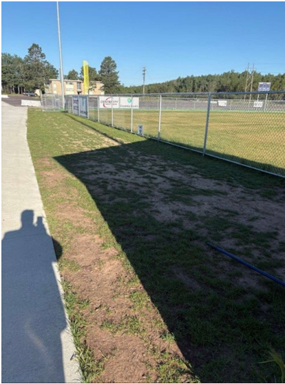
AREA 12 – REPLACE WITH SOD
