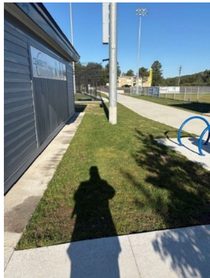
AREA 4 – REPLACE WITH SOD
