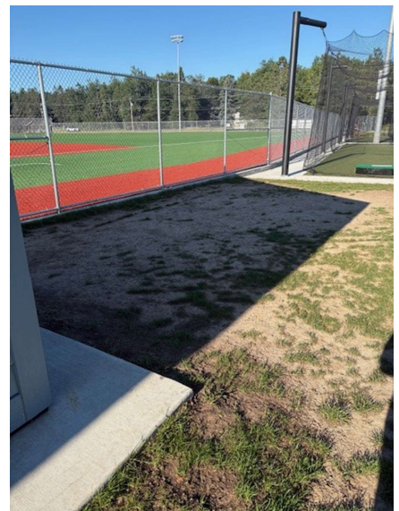
AREA 5 – REPLACE WITH CONCRETE
