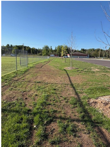
AREA 23 – REPLACE WITH SOD
