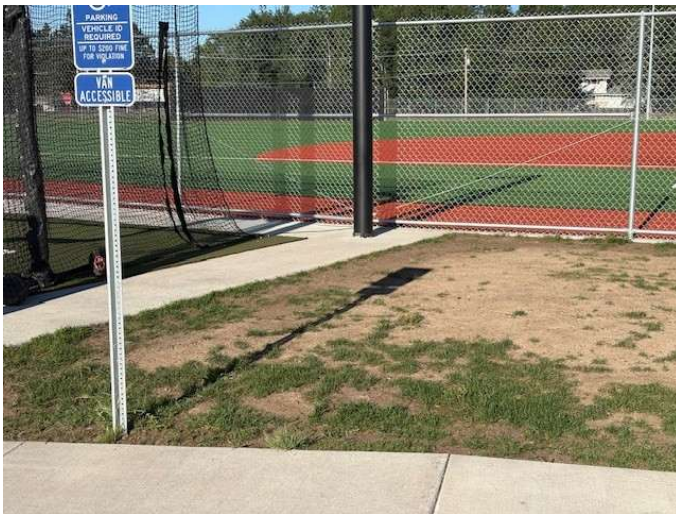
AREA 2 – REPLACE WITH CONCRETE
