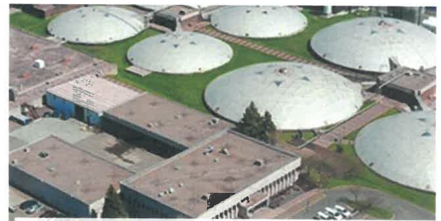
WLSSD Wastewater Facility
